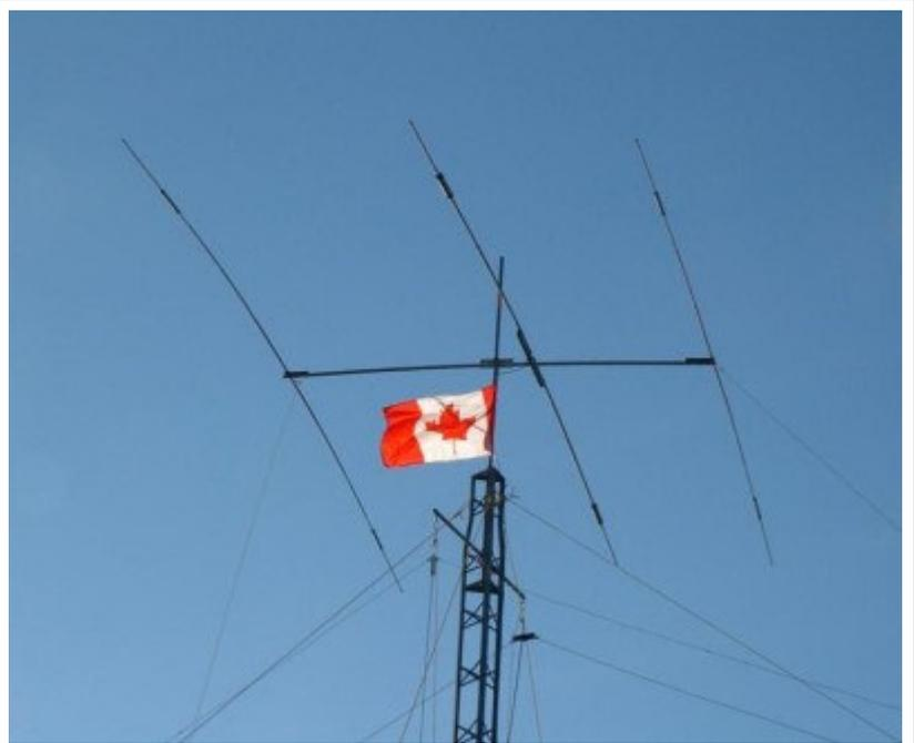
**Fig. 10.7A.1** *Practical implementation of Yagi antenna*
