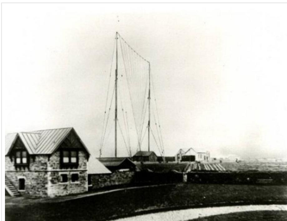
**Fig. 10.1A.2** *Quarter-wavelength dipole antenna of Marconi*
